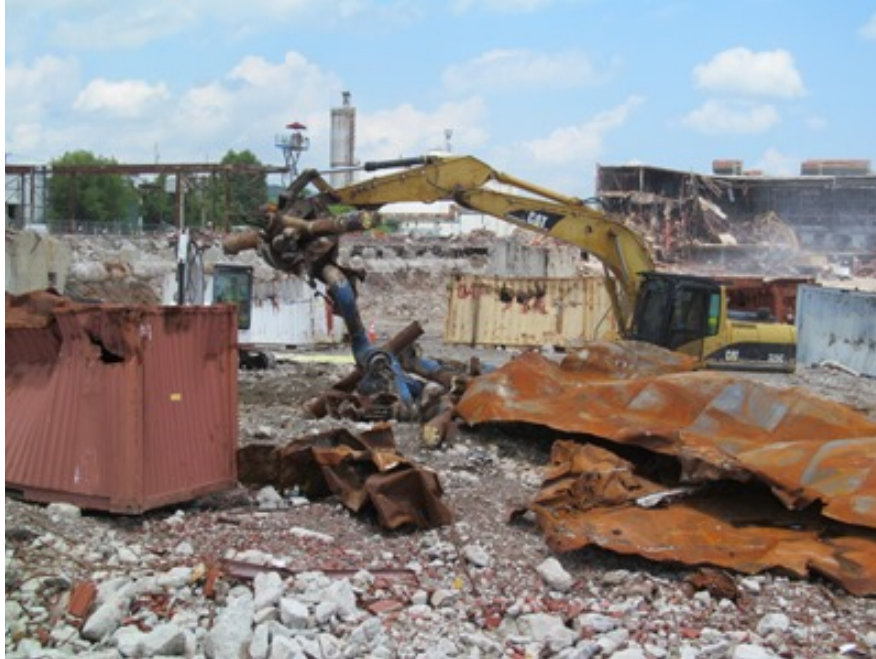
Fig. 3. Special handling of process piping and equipment.
