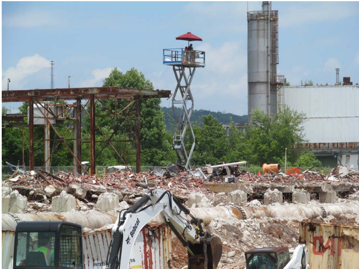
Fig. 4. Spotters overseeing the demo field and monitoring each piece of heavy equipment.
