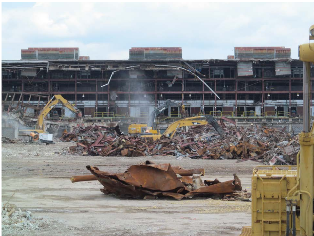
Fig. 2. Demolition equipment operating in the demolition field with continuous water misting being used for dust control.
